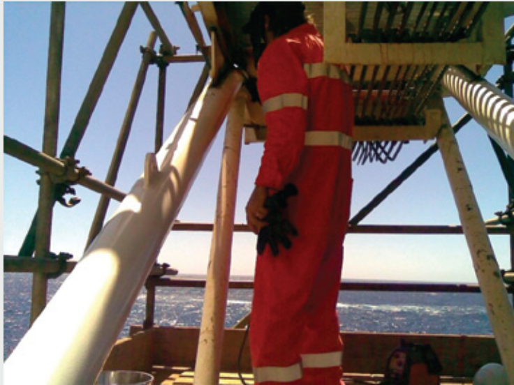
WINNING PHOTO: Welding in an offshore environment. By David Gillespie.
