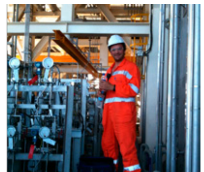
Robert Fishwick commissioning the Chemical Injection Skid
